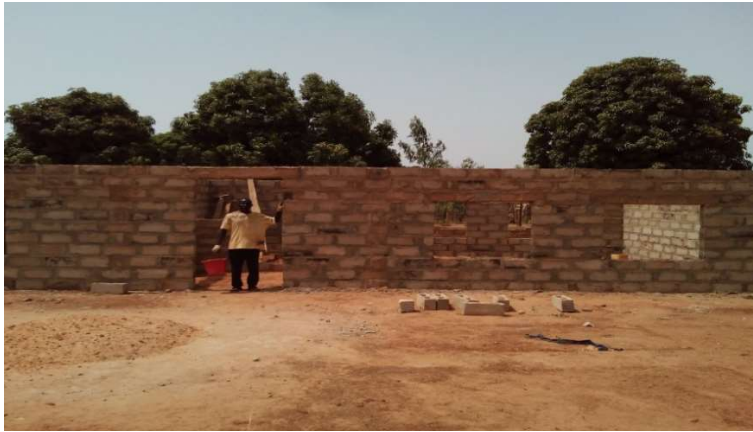
Under construction: POULTRY FARM in Kerewan
